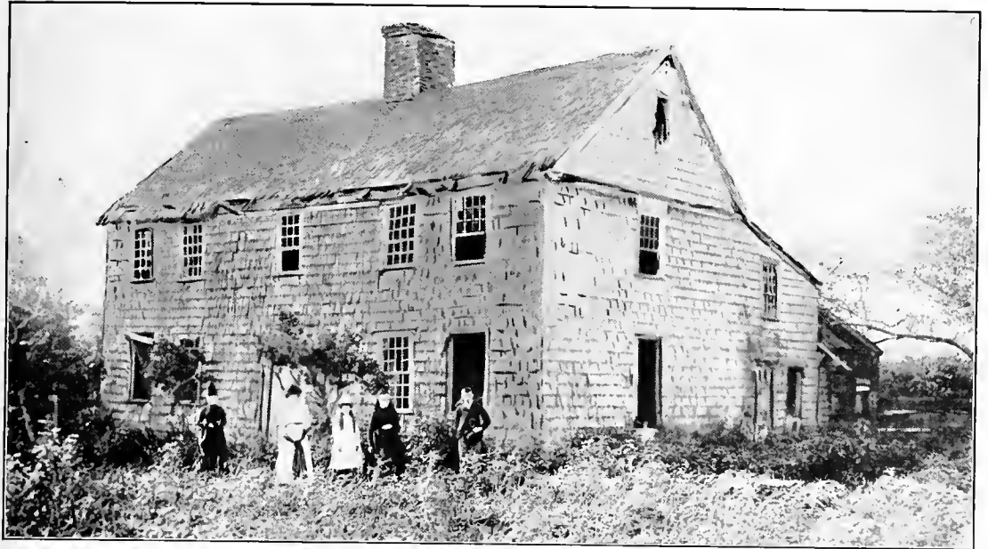
MOSES WHEELER HOMESTEAD, BUILT BEFORE 1700
